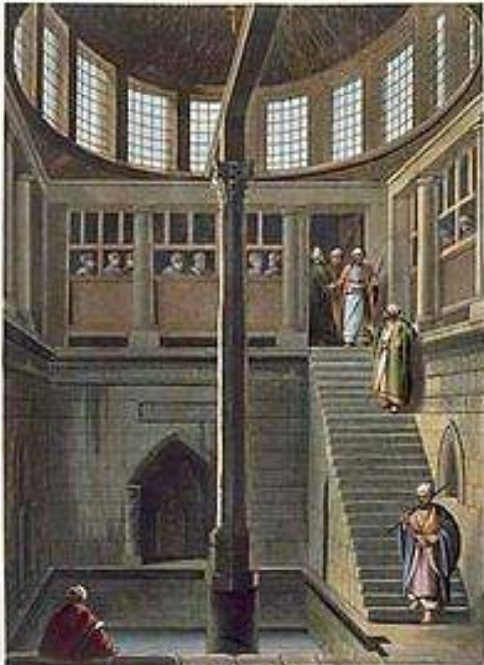
VIEW OF THE TILGHETEN
